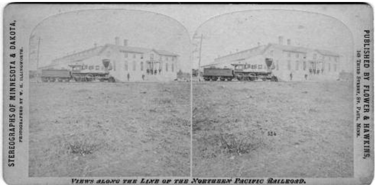
c. 1870's NPRR Repair Shops
